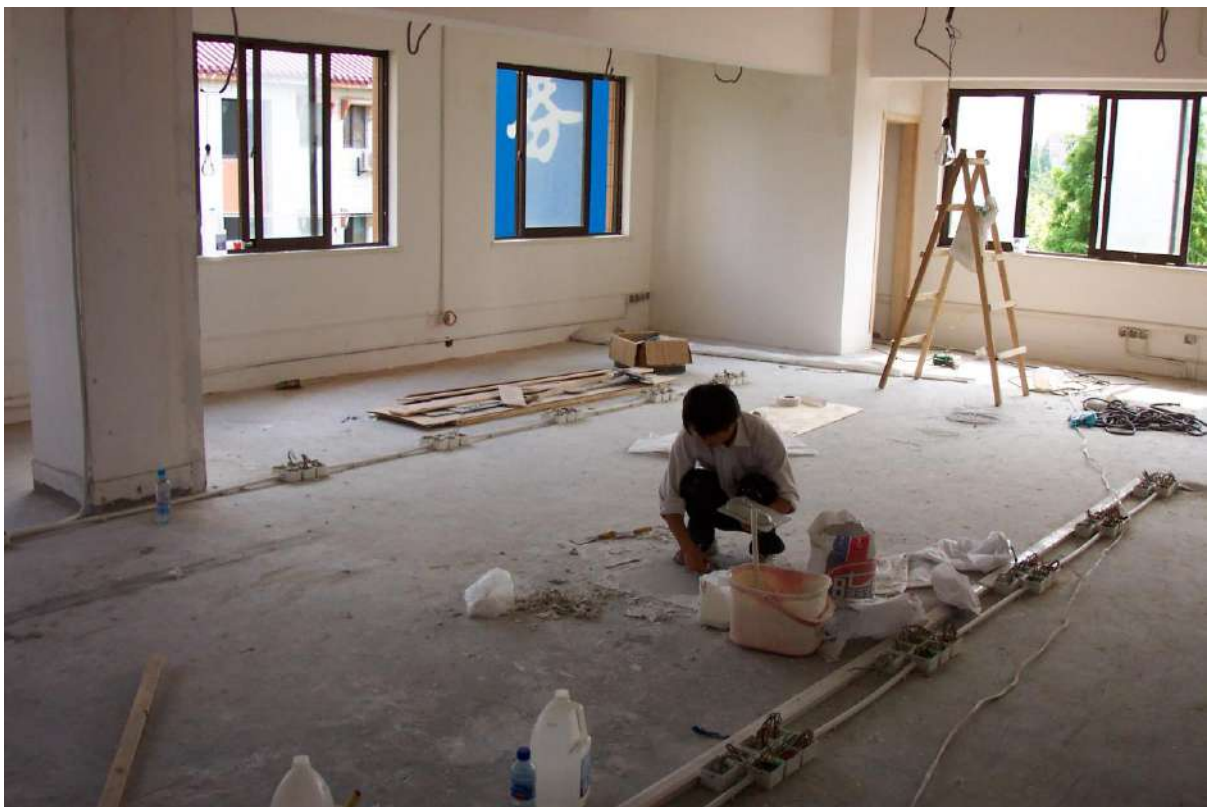
Beginning the build of the photo restoration facility in Shanghai
