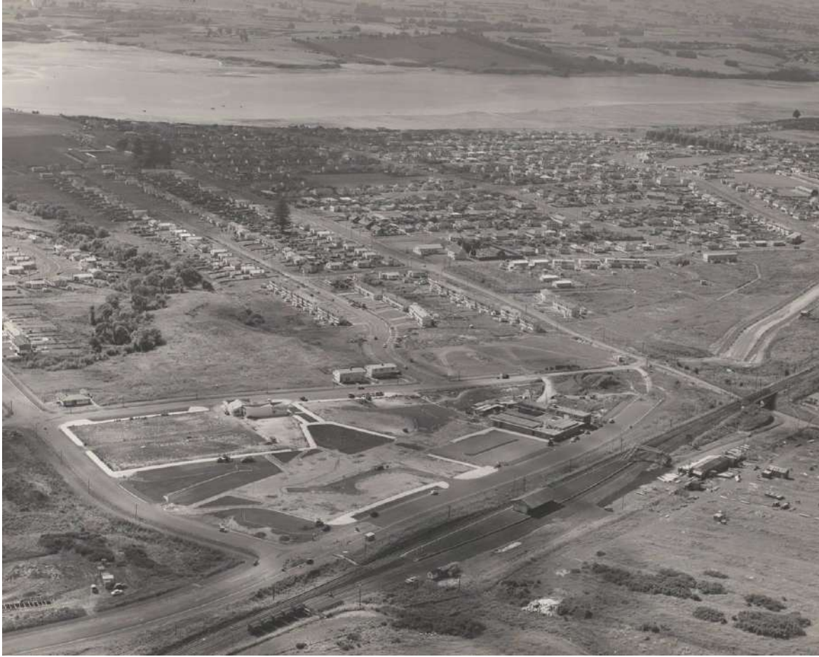
Glen Innes 1959 showing construction of Glen Innes Shopping centre
