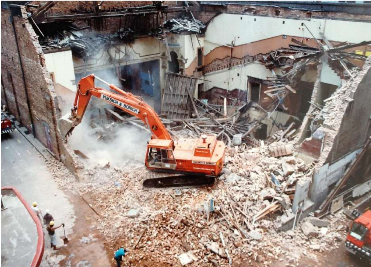
The demolition of His Majesty's Theatre - 1987
