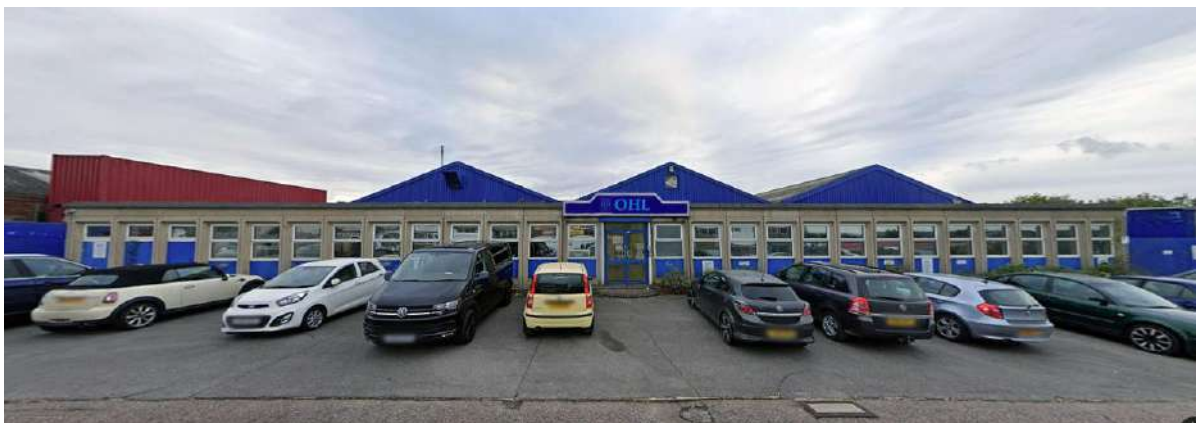
OHL - Lincoln Road, Cressex Industrial Estate, High Wycombe
