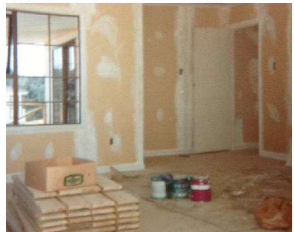
The plastering complete!
